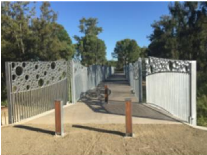
The completed Toogoolawah pedestrian bridge
