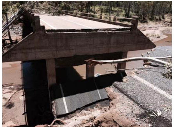
Damage to the eastern abutment of Collard's Creek Bridge following Tropical Cyclone Marcia
