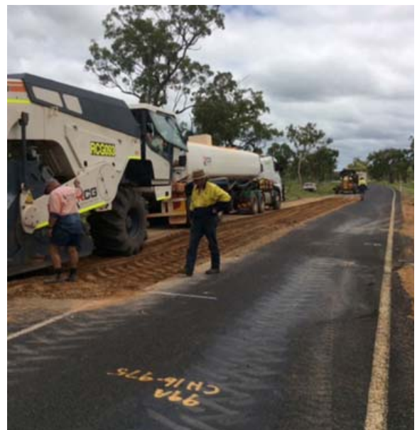
Kennedy Developmental Road – commencing pavement stabilisation
