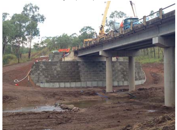
Damage to the eastern abutment of Collard's Creek Bridge following Tropical Cyclone Marcia
