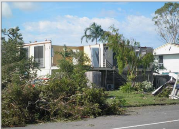
Images above show damage to properties as a result of the recent storm in Townsville (courtesy DARMsys™ team)
