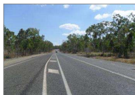
Above: Peak Downs Highway – completed section.
