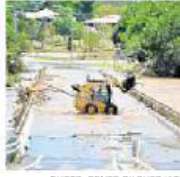
PHOTO: RENEE PULCHER/APM BRIDGE TOO FAR: Normanby bridge under repair.
