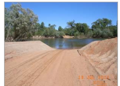
Above: high water level at Hughes Crossing prior to reconstruction.
