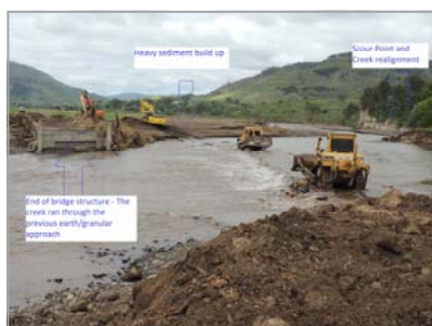
Above: Showing the impact to Hahns Crossing at the bridge and near re-opening (March 2013)
