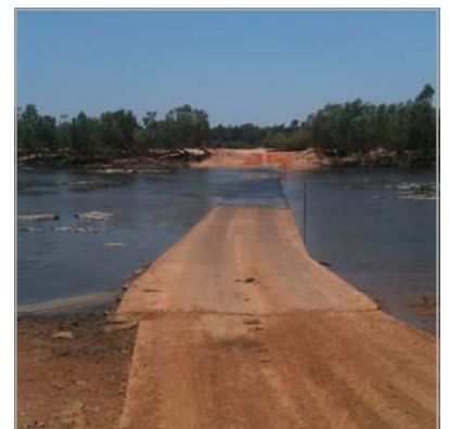
Above: low water level immediately before reconstruction began.
