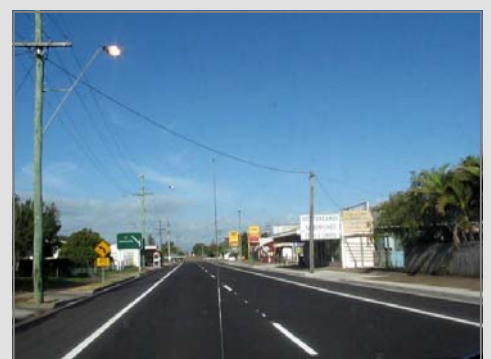
Above: Completed works, seen from a passing vehicle
