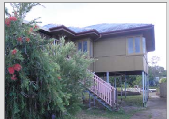
Below: Thanks to Build Back Blitz, it is now fully restored.
