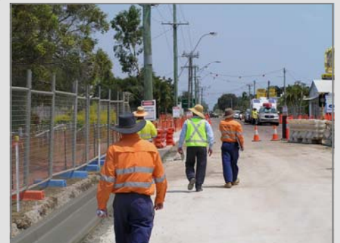
Above: Midway through the reconstruction project
