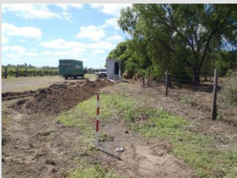
Installation of new gauging station at St George
