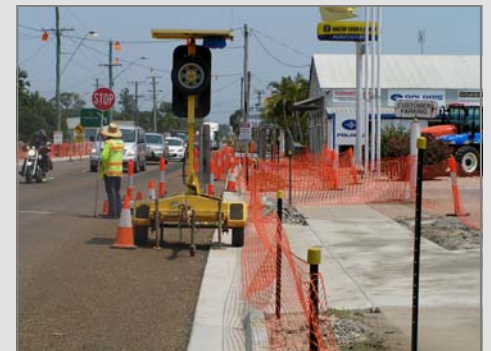
Above: Traffic control on Drysdale Street
