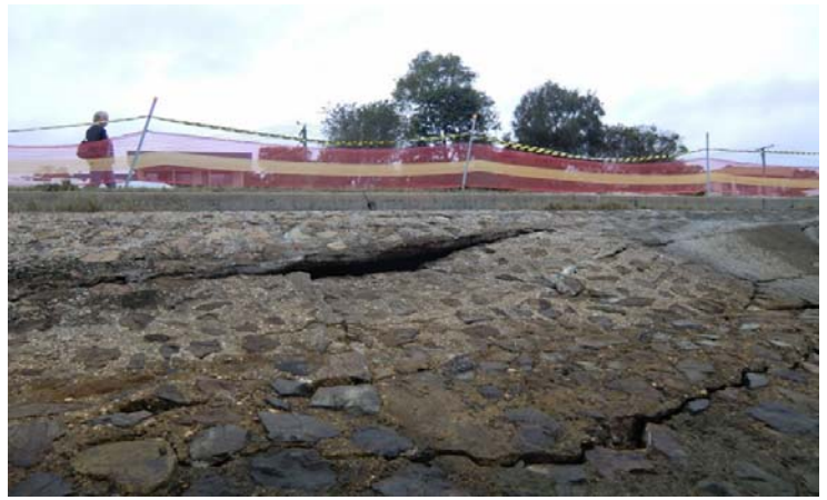
Above: damage to Bongaree Seawall, Bribie Island following storm surges associated with January 2013 disaster event
