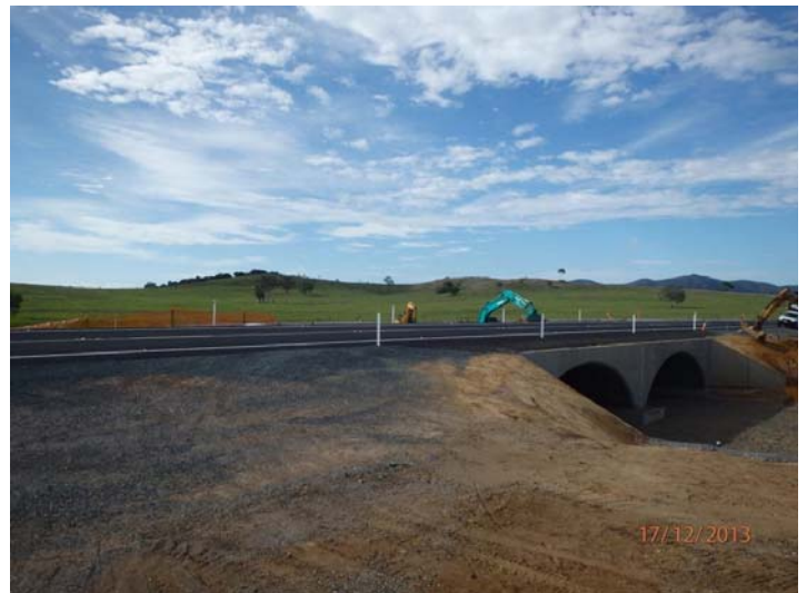
Above: damage to bebo arches culvert structure on Round Hill Road following the 2013 flood event (left); and progress of the works to improve the resilience of the structure, an approved Betterment project
