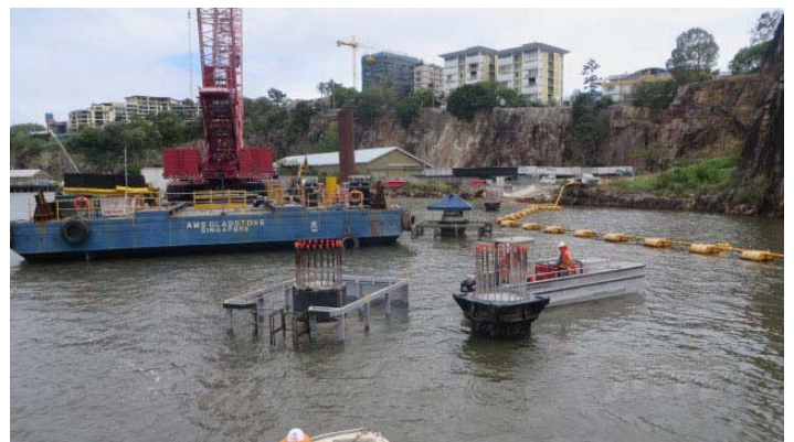
Completed piles on the river
