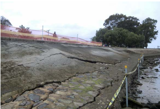
Above: damage to Bongaree Seawall, Bribie Island following storm surges associated with January 2013 disaster event
