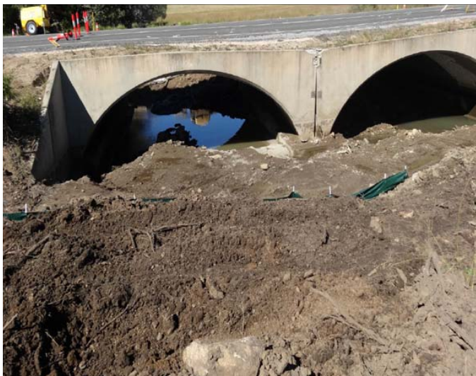
Above: damage to bebo arches culvert structure on Round Hill Road following the 2013 flood event (left); and progress of the works to improve the resilience of the structure, an approved Betterment project
