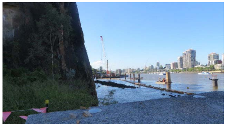
Completed piles showing the future alignment of Riverwalk.
