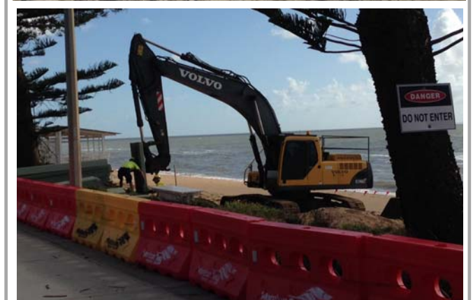
Top: pavement and guardrail damage at the betterment site on Rafting Ground Road, Brisbane City Council
