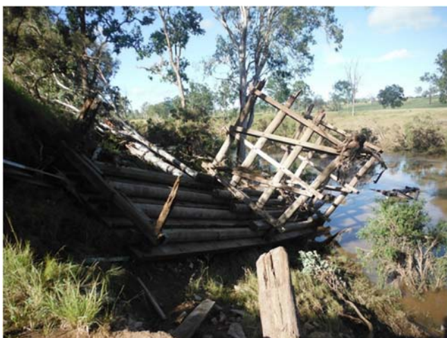
Left: Burnett River Bridge – prior to (top) and following damage (bottom) caused by Tropical Cyclone Marcia in February 2015
