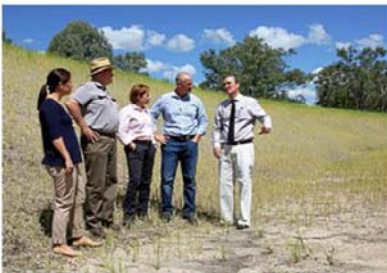
PROGRESS UPDATE: Cr Megan Daniels, Cr Paul Bell, Deputy Premier Jackie Trad, Assistant Minister Glenn Butcher and Mayor Kerry Hayes inspect the completed Nogoa River excavation works. PHOTO: HAYDEN THOMSON CHRC
