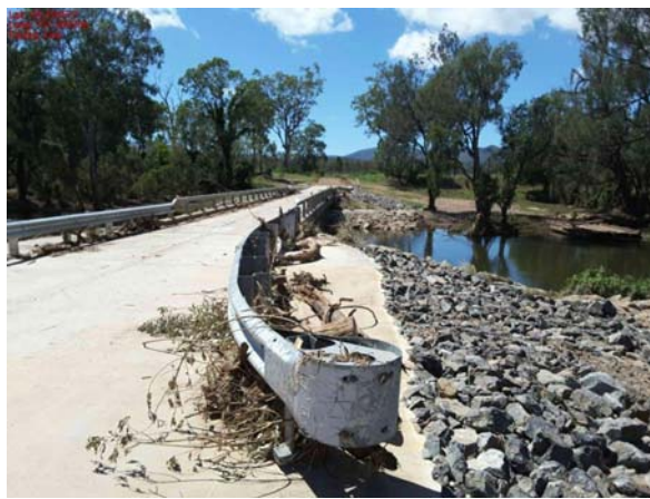
Above: damage to Pilbeam Drive following Cyclone Marcia in 2015 (top); following Betterment works to make the road more resilient (middle); and following Severe Tropical Cyclone Debbie, the site has suffered minor landslip damage only (bottom).
