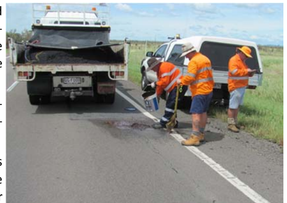
TMR crew pothole patching and updating RADAR in Fitzroy District
