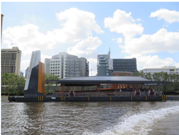
The completed QUT Gardens Point ferry terminal
