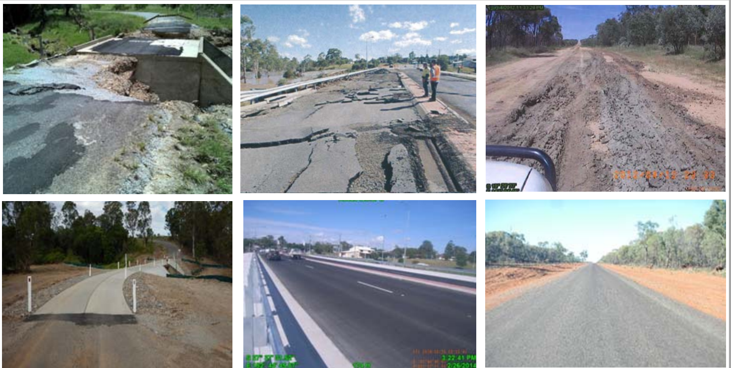
Projects undertaken with Betterment funding — event damage (top) and post completion of works (bottom) - (left to right): Cherry Tree Road (Fraser Coast Regional Council), One Mile Bridge (Ipswich City Council), Richmond Road (Croydon Shire Council)
