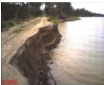
A section of Browns Road (North Burnett Regional Council) washed away following the 2013 floods (above); and the completed realigned road (right)
