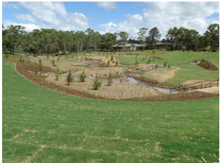
Completed works - Garnet Lehman detention basin
