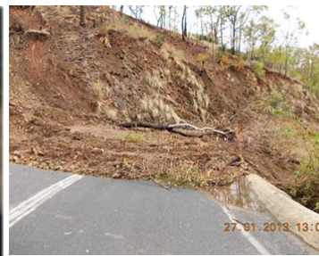
Landslips and damage to the Burnett Highway (Mount Morgan Range) following Tropical Cyclone Oswald (left); and following reconstruction works (right)
