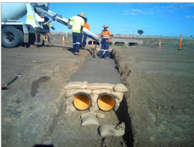
Above: Pouring stabilised sand on side-track drainage beside Landsborough Highway, April 2013.
