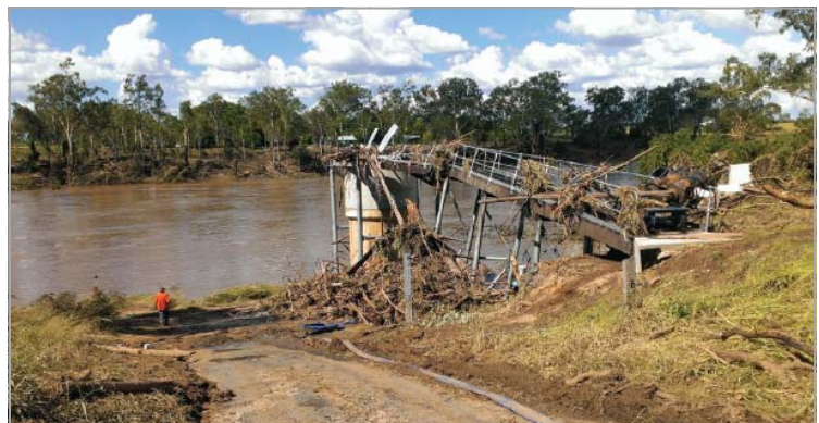
Above: showing extent of redamage to the Gayndah Water Intake Plant in January 2013.
