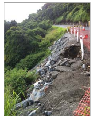
Above: Beechmont Road – landslide below the road near Mirani Street, April 2012
