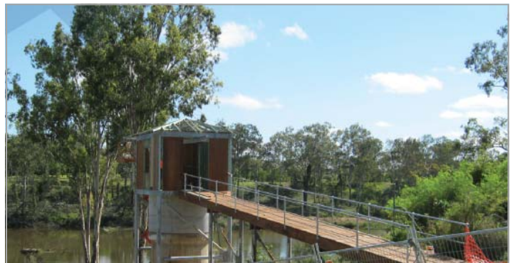
Above: Gayndah Water Intake Plant repaired post 2011.
