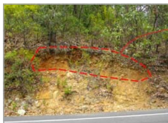
Images above showing damage to slopes along sections of the Captain Cook Highway.
