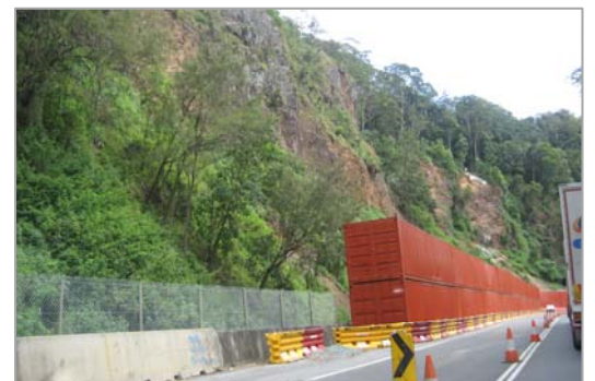
Above: Cunningham's Gap – gravel filled containers and works November 2011.
