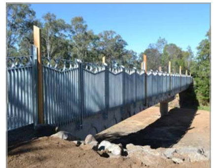
Below The new Esk Pedestrian Bridge
