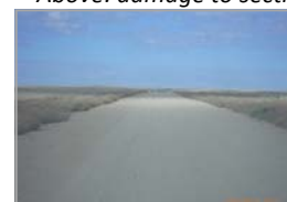
Above: completed sections of Tanbar Road - 2011
