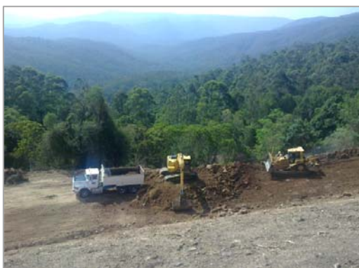
Above: Beechmont Road – reconstruction of landslide, October 2012
