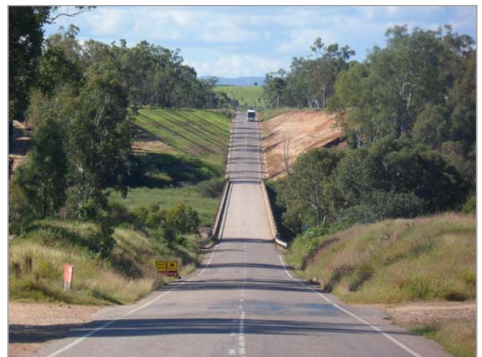
Above: Bowen Development Road - Bowen River batters, right side awaiting hydro-seeding, April 2013.
