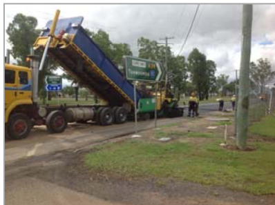
Above: Gore Highway – asphalt work in Millmerran, May 2013
