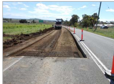
Above: Gore Highway – profiling work near Westbrook, May 2013
