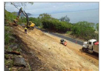
Above: Captain Cook Highway - slope stabilisation works in progress.
