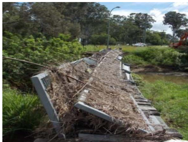
Above: Peak Crossing Pedestrian Bridge, Scenic Rim Regional Council
