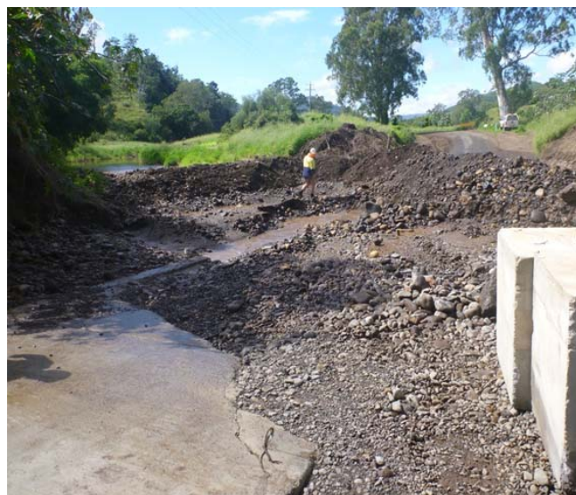
Above: The Left Hand Branch Road floodway, Lockyer Valley Regional Council, completely destroyed by the 2013 floods
