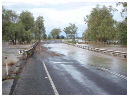
Right: Condamine River Crossing (Millmerran Centenary Bridge) under flooding in 2011 (left) and during works in December 2013 (right).
