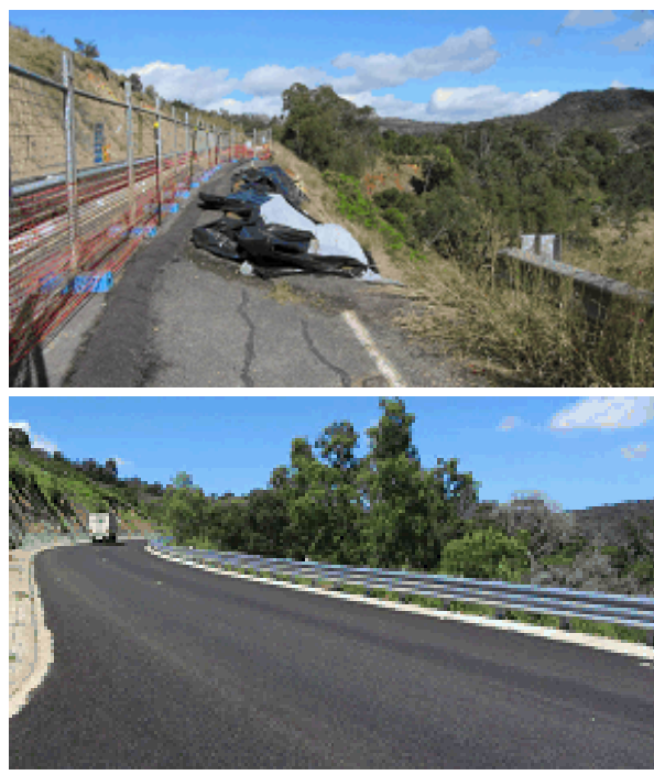
Right: damage to Gatton-Clifton Road (top); and opened to two lanes prior to line marking (bottom) - November 2013
