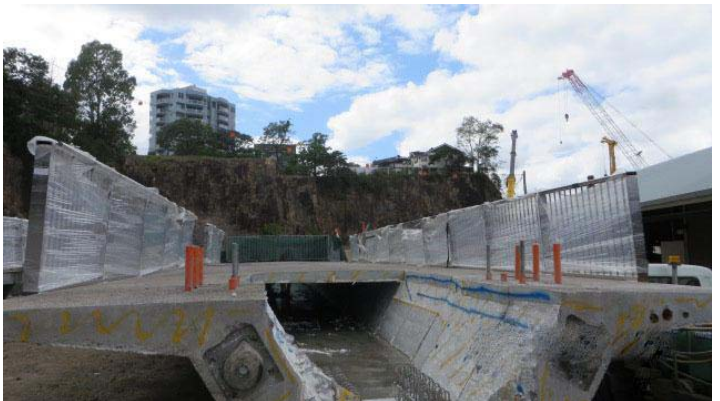
Below right: A prepared pre-cast concrete girder ready for installation
