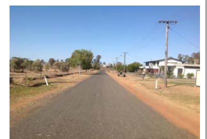
Top: Bundaberg under flood—January 2013 Centre top: damage to Don Tallon Bridge, Bundaberg following 2013 flood event Centre below: completed works Orientos Road, Bulloo Shire Bottom: Completed works—Roma
