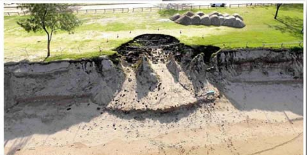
DRONE: Aerial view over Lambert's Beach after Cyclone Debbie. PHOTO: MICHAEL KENNEDY, CHIEF OPERATOR NATIONAL DRONES MACKAY
