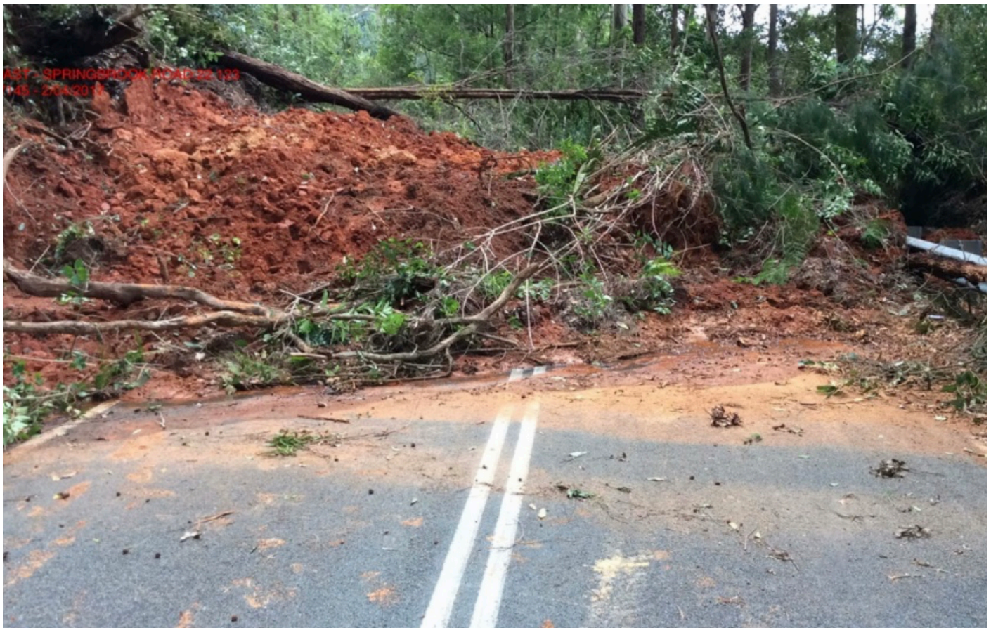
Gold Coast–Springbrook Road – landslide caused by STC Debbie (April 2017)
