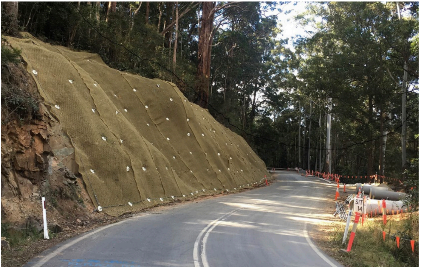
Gold Coast–Springbrook Road – completed soil nail repairs to landslip
