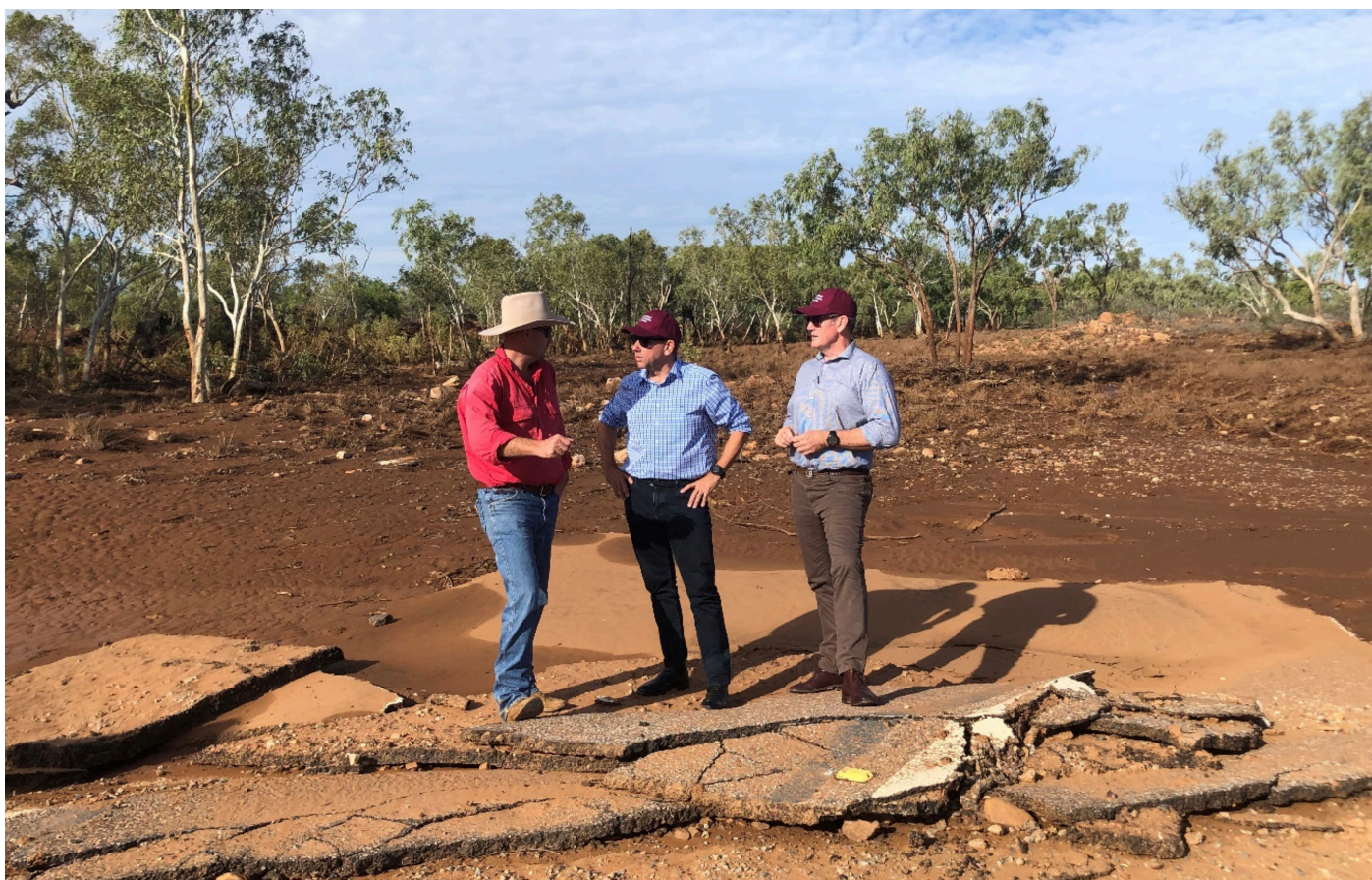
In the aftermath of the floods, Minister Cameron Dick and QRA CEO Brendan Moon travelled to inspect the damage in Cloncurry meeting with Mayor Gregory Campbell
