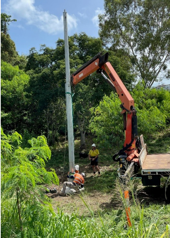
Image: Installation of a flood warning camera asset in Airlie Beach.
