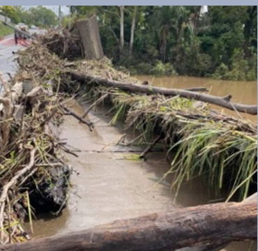
Images above: Granville Bridge – floodwater debris and damage to balustrade and rail.
