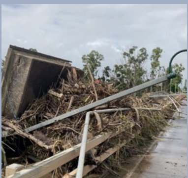
Images above: Granville Bridge – floodwater debris and damage to balustrade and rail.
