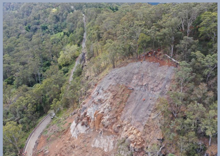
Image: Tamborine Mountain Road – mesh and rock dowel works
