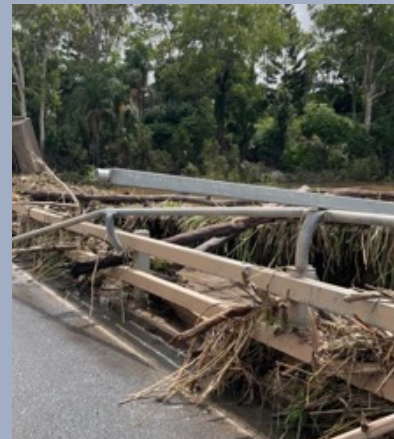
Images above: Granville Bridge – floodwater debris and damage to balustrade and rail.
