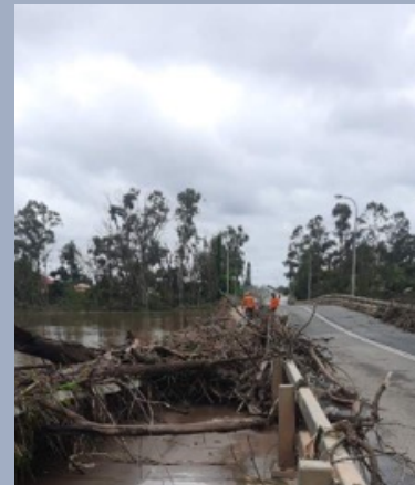
Images above: Granville Bridge – floodwater debris and damage to balustrade and rail.
