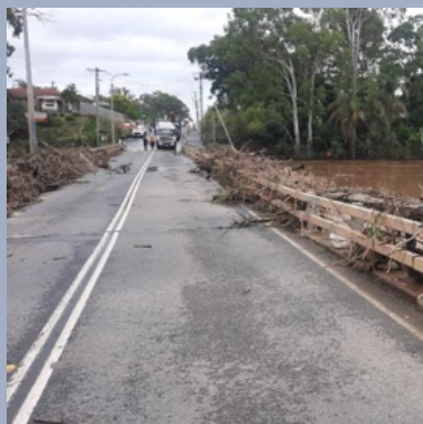
Images above: Granville Bridge – floodwater debris and damage to balustrade and rail.
