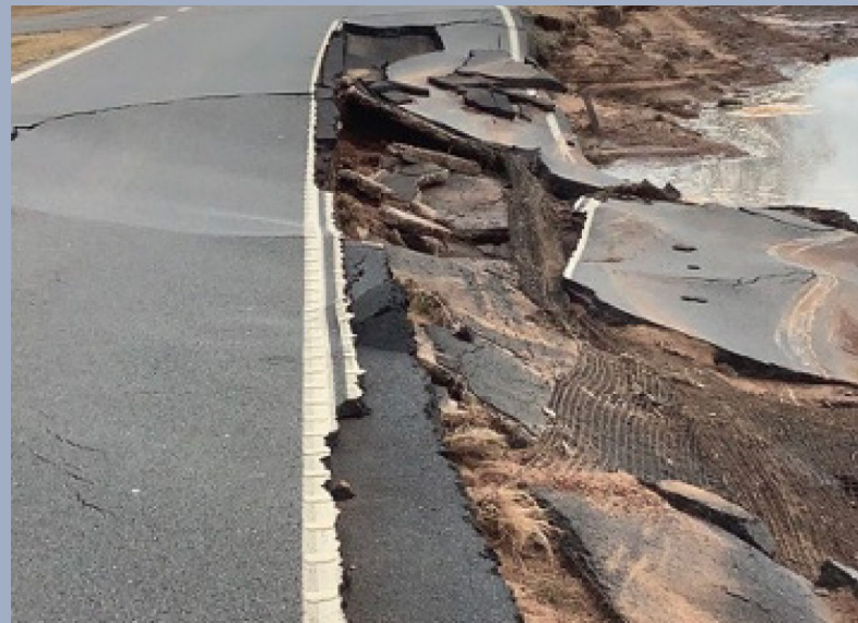
Images: Brisbane Valley Highway (Ipswich–Harlin) at Geoff Fisher Bridge – damage from SEQ Rainfall and Flooding
