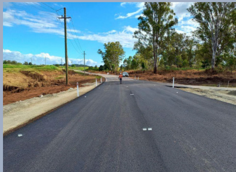
Image: Completed emergency works.
