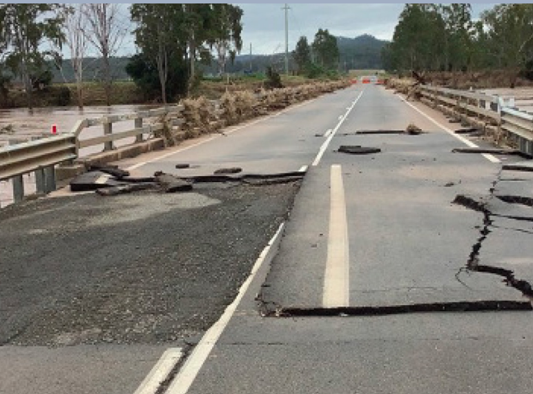
Images: Brisbane Valley Highway (Ipswich–Harlin) at Geoff Fisher Bridge – damage from SEQ Rainfall and Flooding
