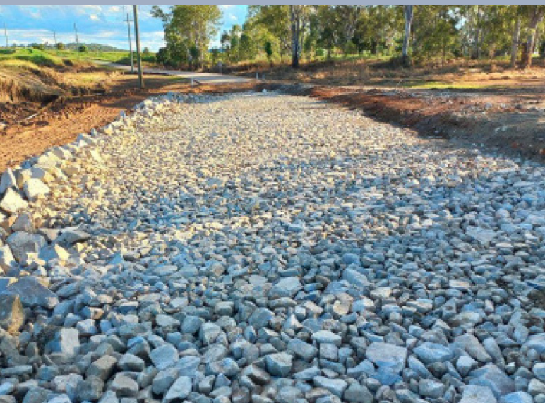
Image: Rock base installed.
