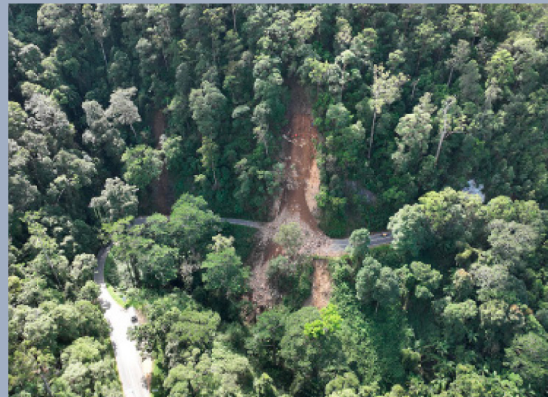
Image: Gold Coast–Springbrook Road – landslip following heavy rainfall in late March 2022.
