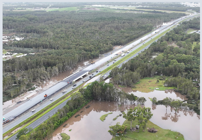
Bruce Highway looking south towards King John and Lagoon Creeks (February 2022)
