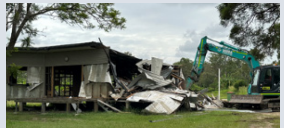
Demolition crews at work removing flood-vulnerable houses in Goodna – January 24, 2023
