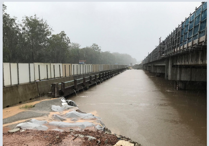
Bruce Highway – new and old bridges at Six Mile Creek (February 2022)
