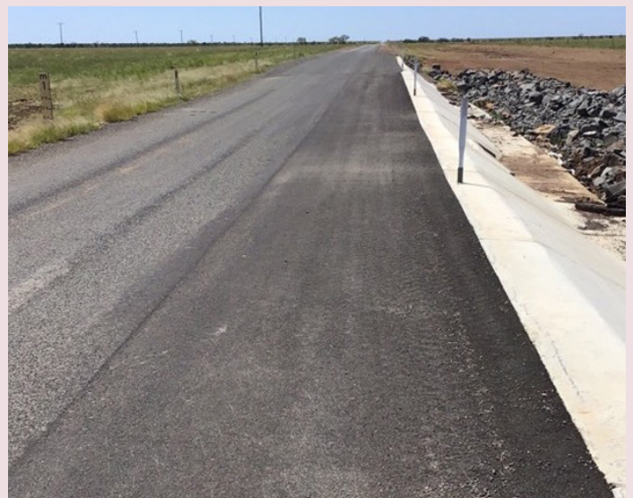
Muttaborra–Aramac Road – completed reconstruction works (October 2022)
