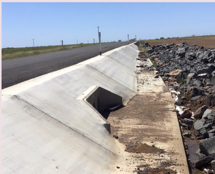
Muttaborra–Aramac Road – completed reconstruction works (October 2022)
