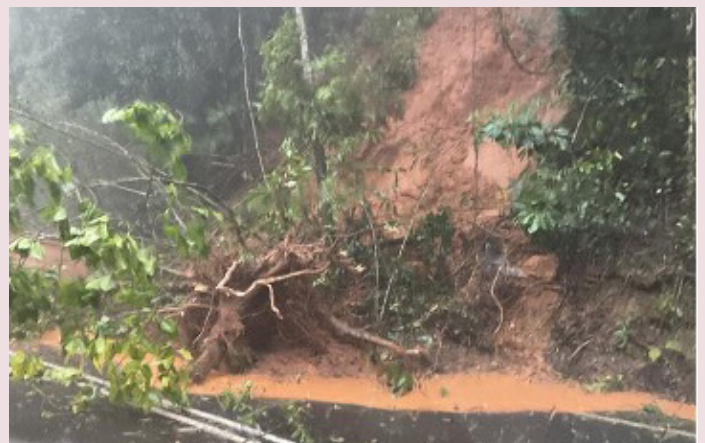
Kuranda Range Road – landslide (December 2023)
