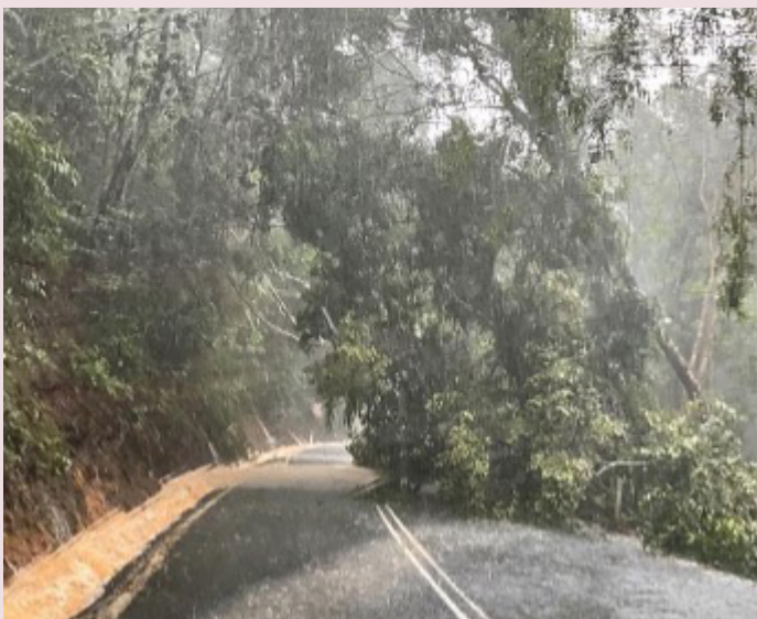
Kuranda Range Road – fallen vegetation (December 2023)
