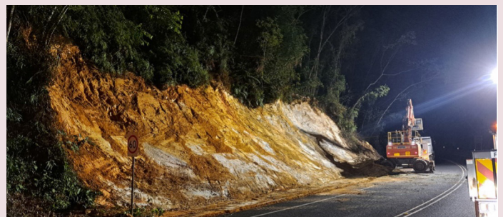
Kuranda Range Road – night works (January 2024)
