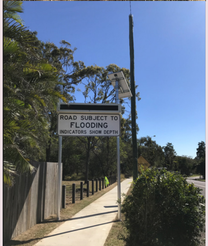
Examples of FWIN in Queensland: (top) An automatic River Height Camera; (bottom) Automatic Flood Warning Road sign
