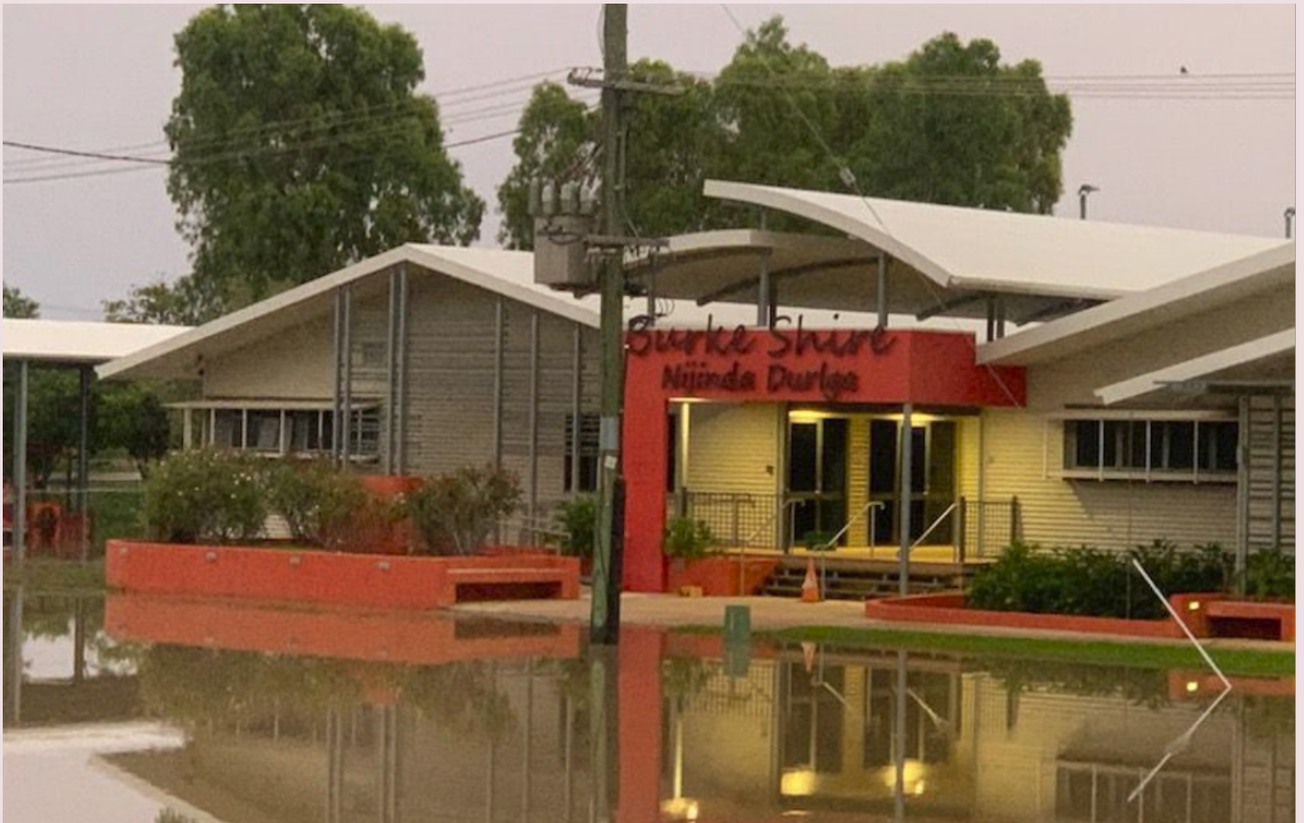
Floodwaters from Tropical Cyclone Kirrily lap Burke Shire Council buildings
