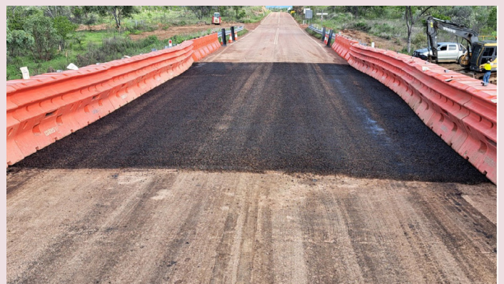
Gulf Developmental Road at Routh Creek Bridge – completed
